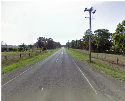
Figure 2.5: Hollinsworth Road (looking west)
